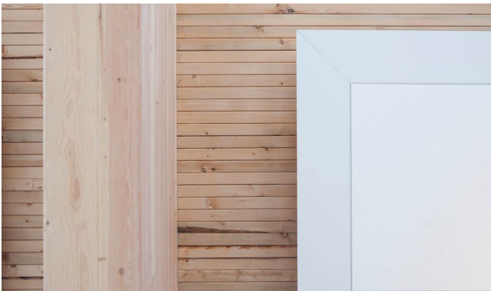
Image 9.3 Glue-laminate beams with pine beetle kill wood decking. Photograph by Enrico Dagostini.
